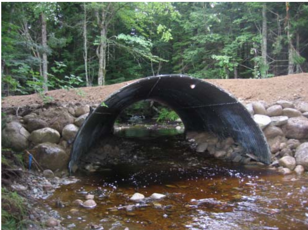
Looking upstream to new 15 ft wide Open Arch. Aug 12, 2011
