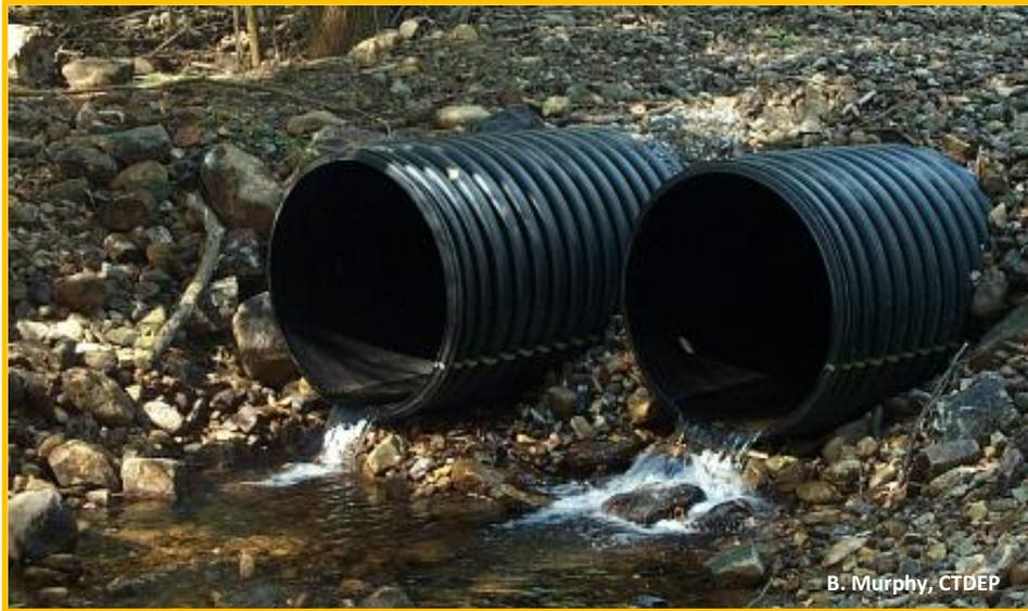
Figure 1. Photograph depicting outlet of twin culverts perched above streambed. Improper culvert installation blocks and prevents upstream passage for the wild brook trout population.
