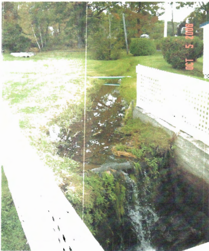
Belfast, Maine: Unnamed Stream, existing dam and view of stream channel. Photograph: W. L. Woodward, Oct, 5, 2006.
