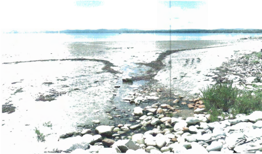
2011: downstream @ low tide, pipes are 100% submerged @ MHW Photograph: R. Van Riper, July 2011
