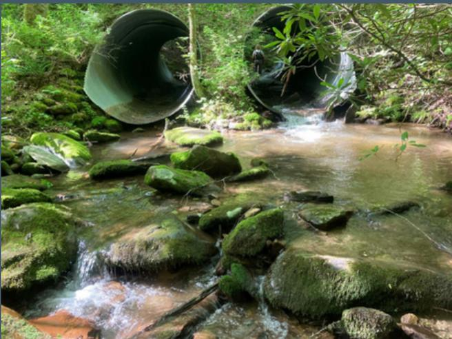
Undersized culverts on Trail Fork of Big Creek will be replaced with a natural-bottom structure that allows for full passage of brook trout and aquatic organisms. This will also connect 2.5 miles of Trail Fork.
