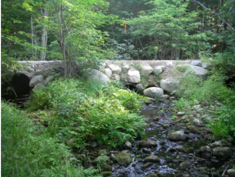
Looking upstream to Old Culverts (n=5).
