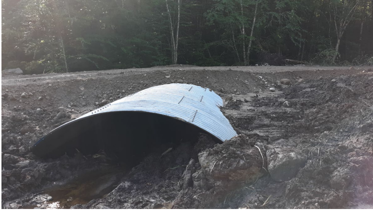
W. Musquash Culvert Project - After
