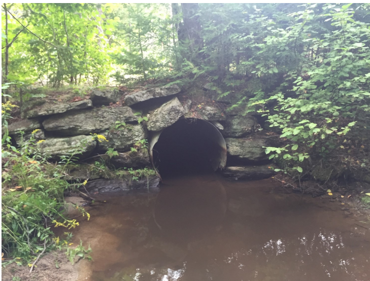
W. Musquash Culvert Project - Before
