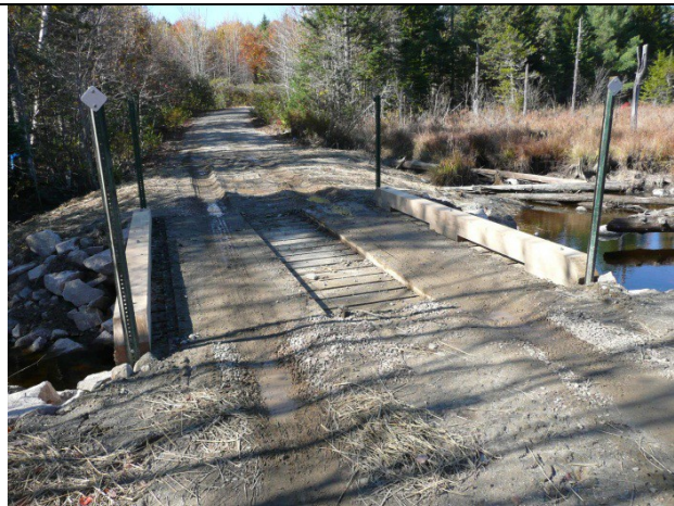
Figure 14: Bridge at site 127.
