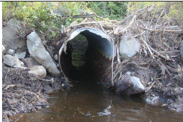
Figure 12: Before - inlet at site 127.
