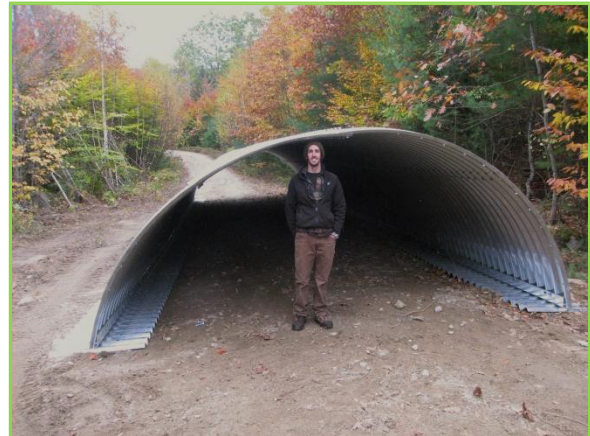
Figure 25: Ash Bog Stream culvert. Photo by Dan Grenier.
