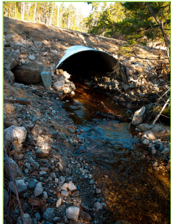
Figure 35: Black Rock Brook downstream following culvert installation. Photo by Nancy Sferra.
