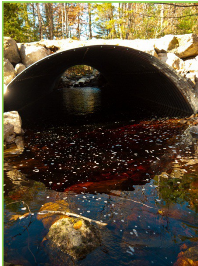
Figure 28: Ash Bog Stream culvert outlet following construction. Photo by Nancy Sferra.
