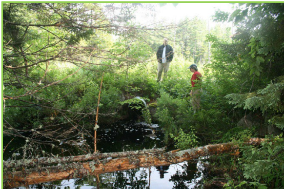
Figure 34: Black Rock Brook upstream of culvert before restoration. Photo by Scott Craig.
