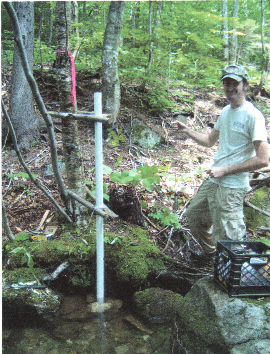
6/27/08. Installation of a stilling well for a water level logger, Sunday River treatment site #2 above chop and drop area. Photograph by Jeff Stern, Androscoggin River Watershed Council.
