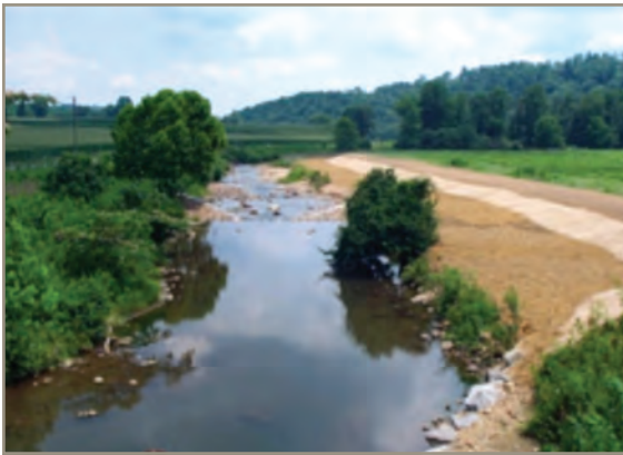
Figure 9.1a Restoration site immediately after construction.
