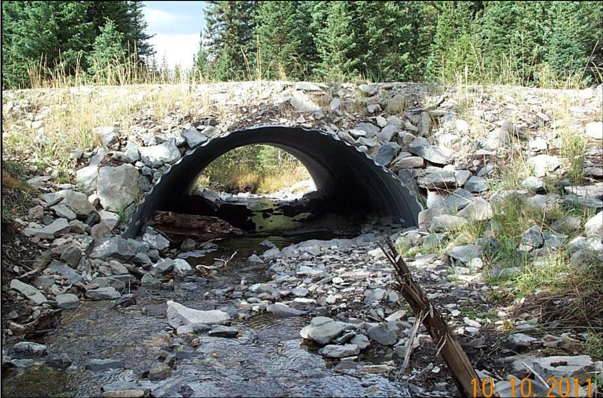
**Figure 2.** Culvert built to mimic natural stream reaches. The stream flow and substrate within the culvert remains similar to that of the adjacent upstream and downstream reaches. In this case fish passage should be assumed.
