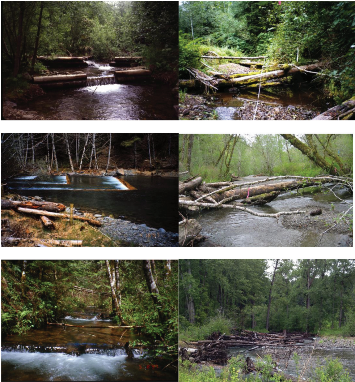
Fig. 2. Examples of common types of wood placement used in North America. Photos on the left represent immobile wood structures commonly used prior to 1990s, although similar designs are still in use today. In contrast, photos on the right show modern techniques using more mobile or natural wood with limited or no anchoring.
